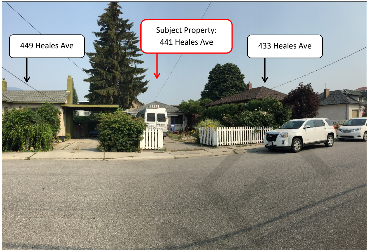
Figure 5 – Looking toward front of 441 Heales Avenue from the street
